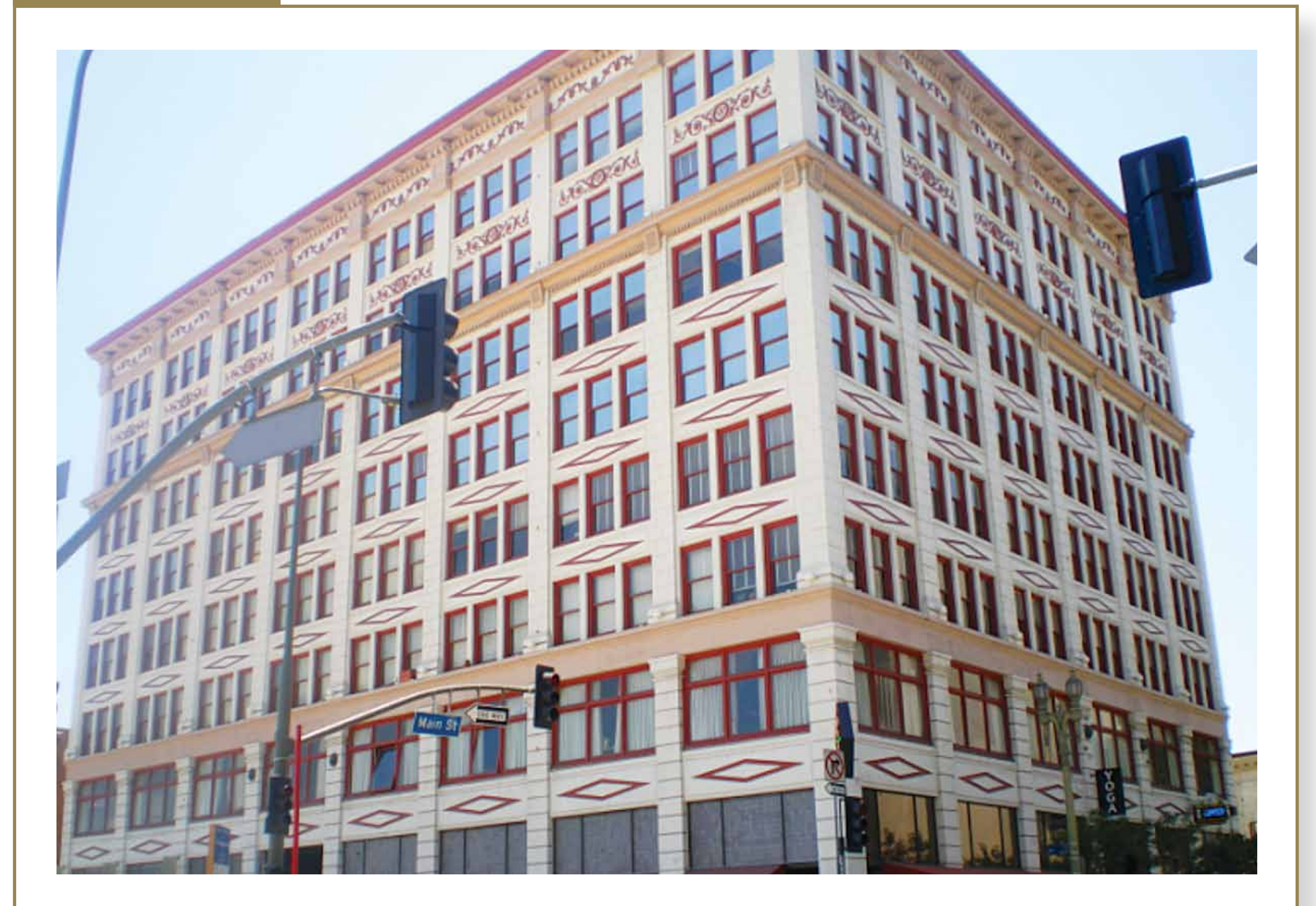
This is an example of an appropriate rehabilitation of a historic structure. The building's form and character defining features have been retained. Its storefronts, storefront bays, and fenestration patterns have also been maintained.
