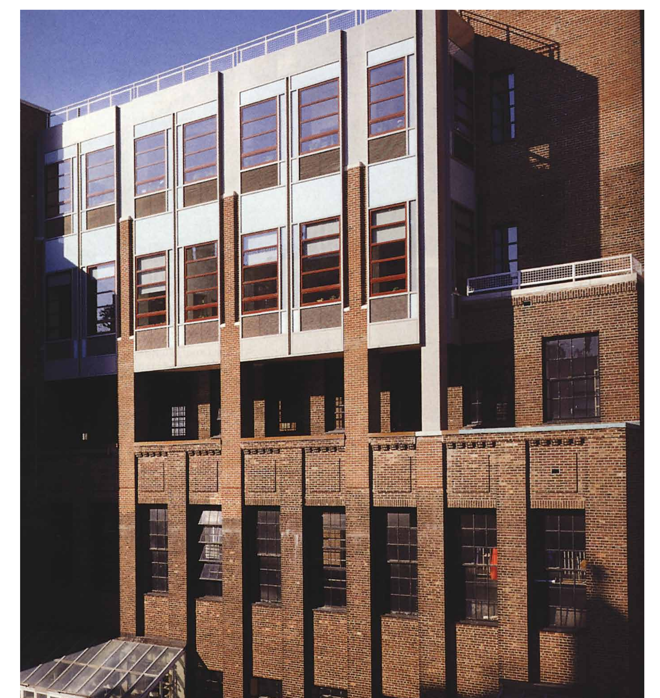
The rooftop addition continues the lines and materials of the original building before transitioning into new materials and forms. This technique creates a more seamless intersection between new and old.
