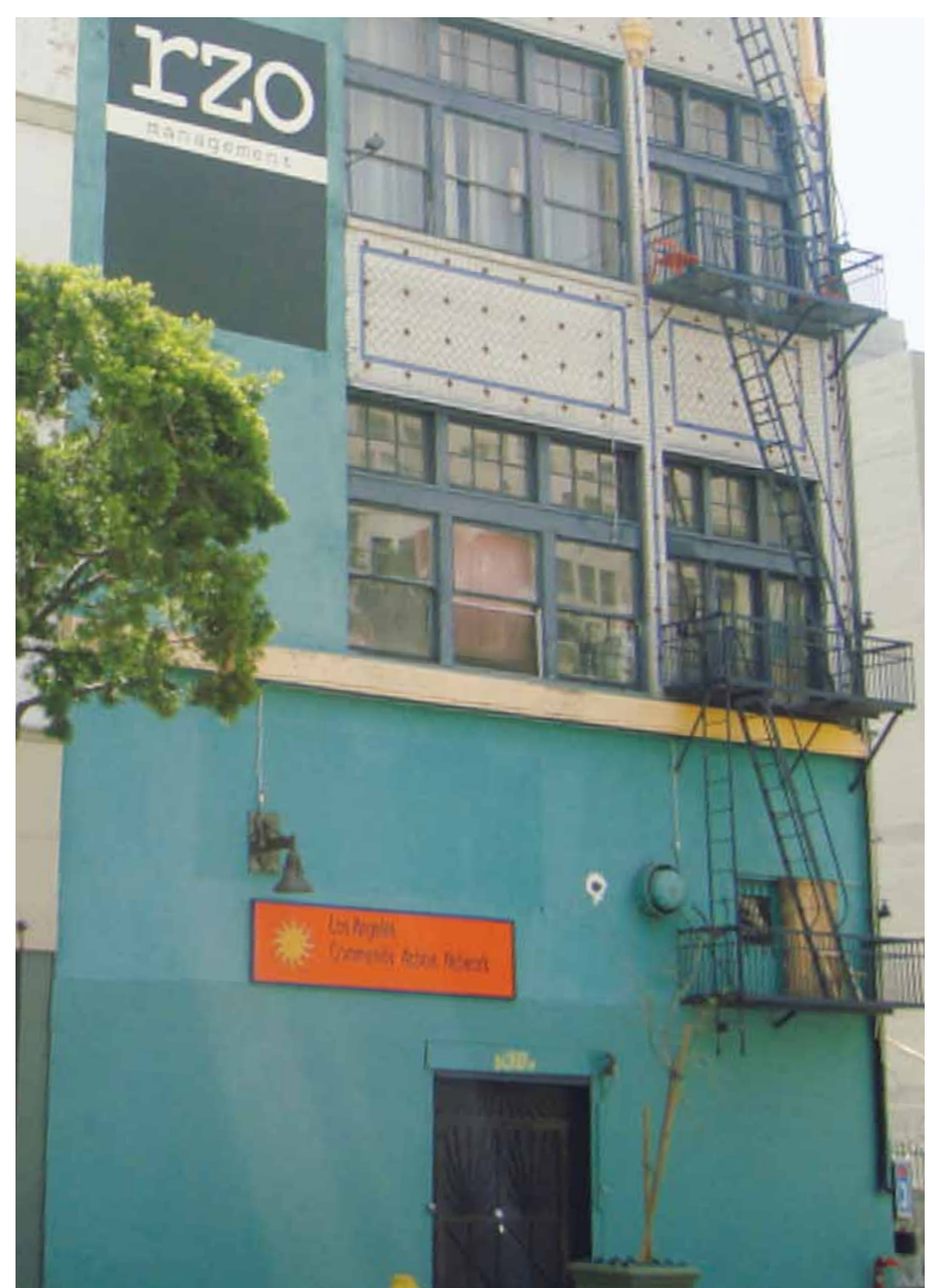
The building lacks transparency and storefronts on the ground floor.
